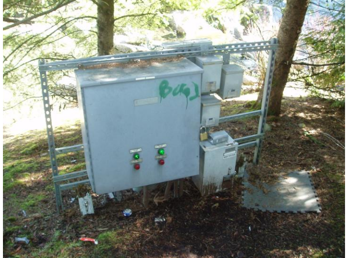
Photo 2. Front view of old control panel showing on/off lights for each pump.
