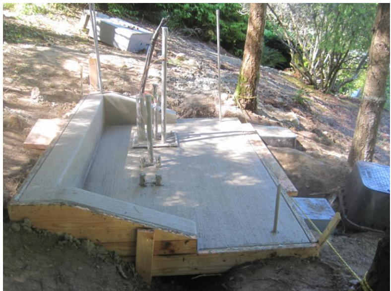
Photo 4. Concrete foundation for new control panel and building.
